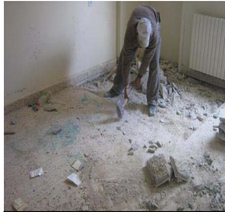
Hospital before the project
