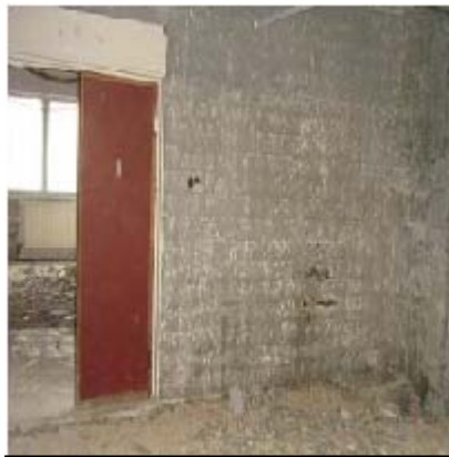
The site before rehabilitation starts
